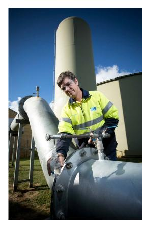
Busselton Water closely manages chlorine dosing levels to maintain a minimum residual chlorine level of 0.4 milligrams per litre throughout the distribution system. During the year, Busselton Water collected 1.244 chlorine samples in the distribution network. The minimum total chlorine level was 0.21 milligrams per litre (in a new street slowly establishing consistent flows) and the maximum was 0.92 milligrams per litre.
